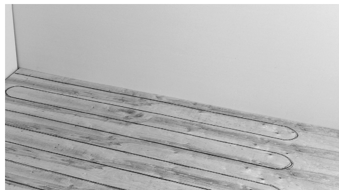
Fig. 11: Mark pipe location before securing underlayments over RAUBOARD to subfloor (if required)
