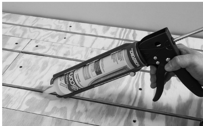
Fig. 15: Apply silicon in grooves
