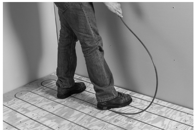
Fig. 10: Install pipe with silicon in groove
