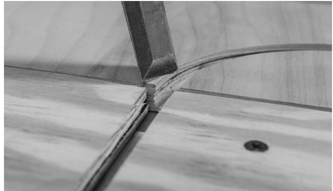
Fig. 8: Re-position panels to align grooves, shaving sharp edges
