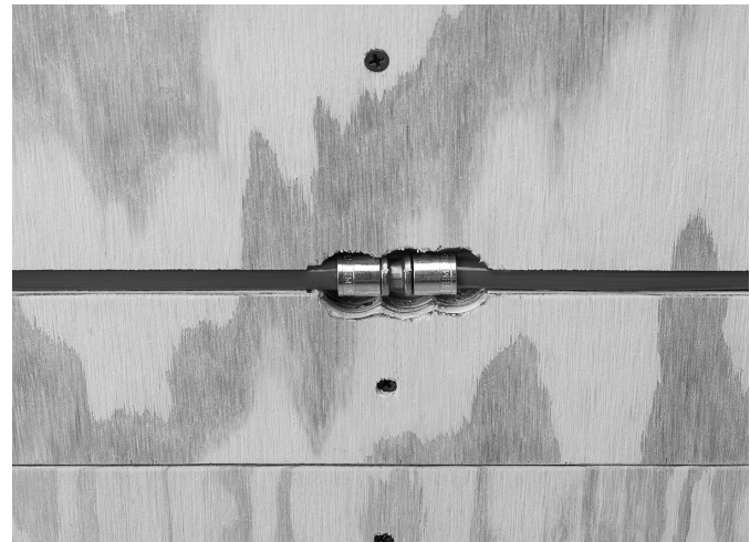
Fig. 21: Replace damaged pipe in RAUBOARD (if required)
