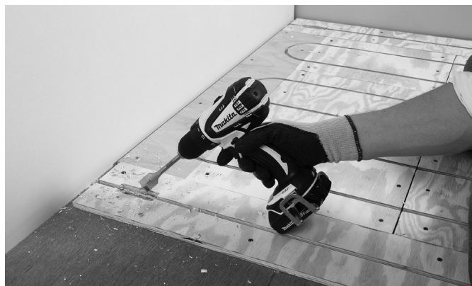
Fig. 14: Drill subfloor penetrations for supply and return tails
