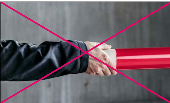
Fig. 03-26 Do not touch the welding areas on the pipe ends. If necessary, clean dirty welding areas with Tangit cleaner again.
