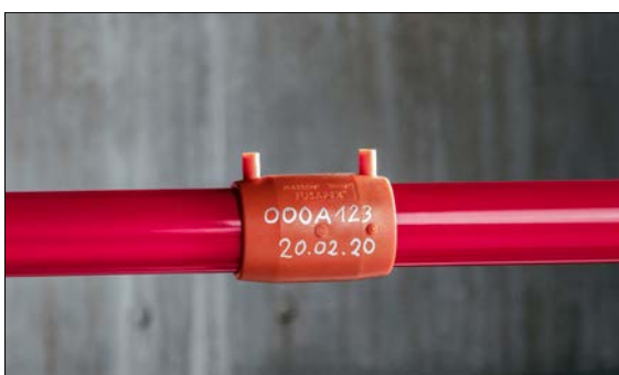
Fig. 03-20 FUSAPEX joint is complete.
