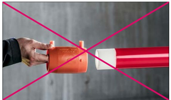
Fig. 03-27 Do not touch welding areas in the electrofusion fitting. If necessary, clean dirty welding areas with Tangit cleaner prior to welding.
