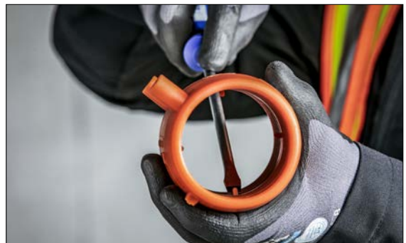
Fig. 03-34 The electrofusion fitting can also be used as a sleeve coupler. To do so, carefully remove the end stop inside.
