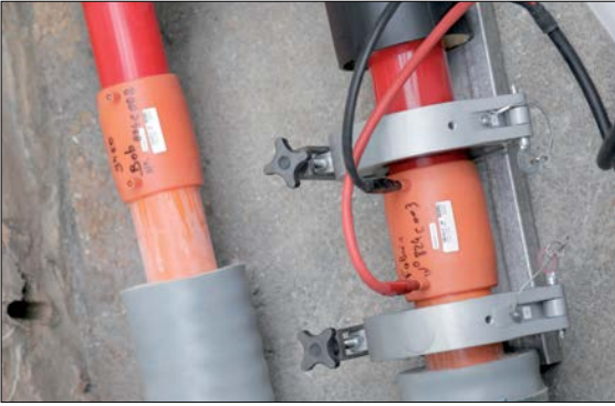
Fig. 03-21 In case of greater positional deviations (e.g. pipe coils), the pipe ends must be pre-aligned with additional pipe bending or holding devices before the pipe retaining clamps are installed.
