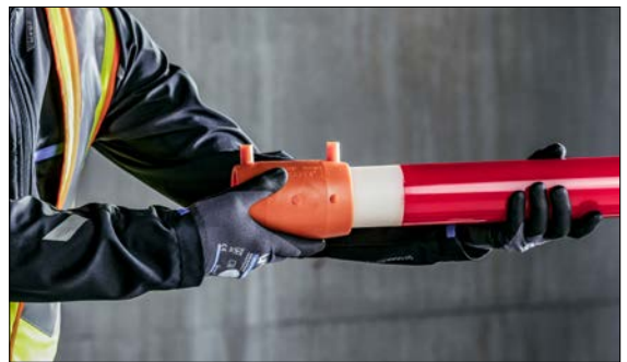
Fig. 03-10 Push the FUSAPEX electrofusion fitting onto the pipe end all the way to the end stop.
