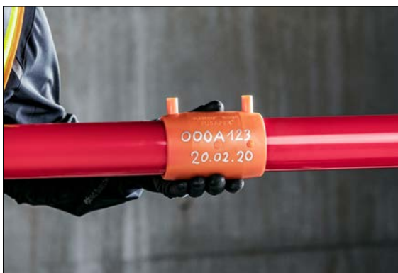
Fig. 03-19 Before commissioning and pressurisation can take place, you must comply with the extended cooling down time in Tab. 03-4.
