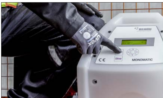
Fig. 03-15 Check the welding parameters in the display and confirm by pressing the start button. Confirm the display again to start the welding process.
