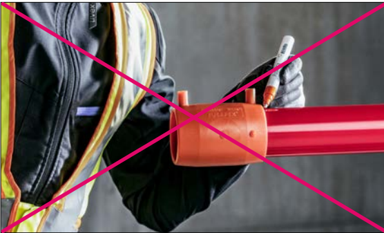
Fig. 03-22 Do not use the electrofusion fitting for marking.
