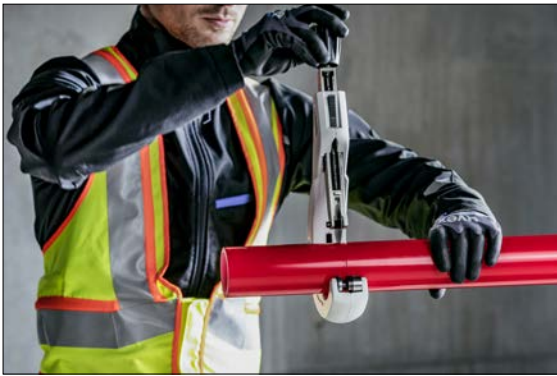
Fig. 03-1 Cut pipe to the required length. The pipe end must be straight, square and free of burrs.
