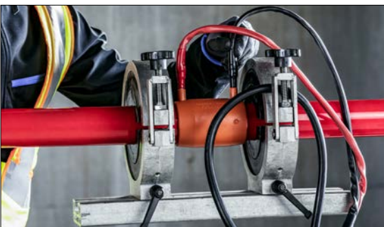
Fig. 03-13 Connect the REHAU welding machine with SMART-FUSE technology (red cable to red contact). The welding parameters are determined automatically.
