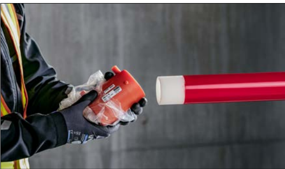
Fig. 03-9 Only remove the FUSAPEX electrofusion fitting from the bag at this point. If necessary, clean the fusion fitting with Tangit cleaner on the inside and let it evaporate completely.
