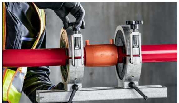
Fig. 03-12 Attach the pipe retaining clamps. The connection must be free of tension during the welding process.
