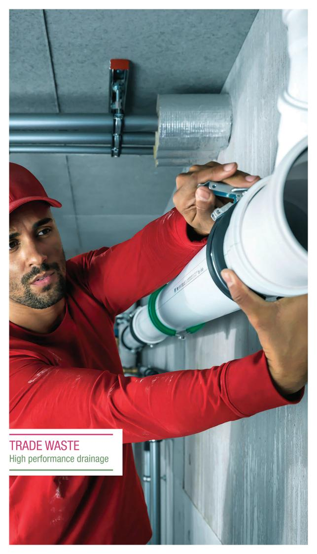
RAUPIANO PLUS is made of mineral reinforced Polypropylene (PP-MD) with high temperature and chemical resistance. This makes it an ideal drainage solution for hot kitchen trade waste.
