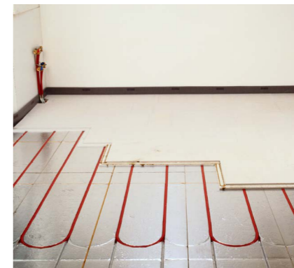
Floating floor Pre-routed polystyrene panel laminated with an aluminium foil. Fast response time but requires a load bearing subfloor.
