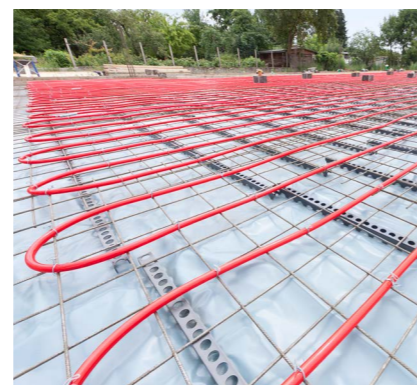
Industrial floor heating Ideal for large warehouses and hangars which are typically harder to heat. Pipe installed directly in the concrete slab using a reinforcement mesh.
