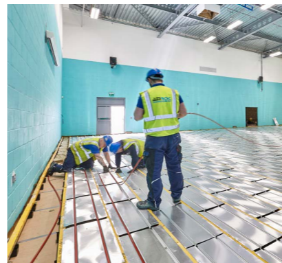
Diffusion plate Designed for timber joist or batten floors such as sports halls. Faster reaction times than screeded systems.
