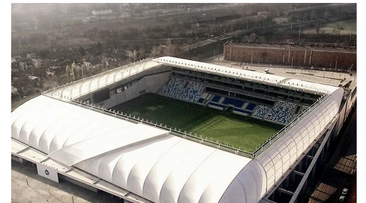
MTK stadium Budapest: 28,000m of pitch heating
