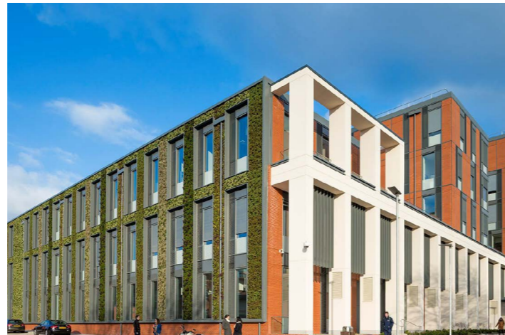
University of Leicester 7,000m of industrial floor heating / TABS
