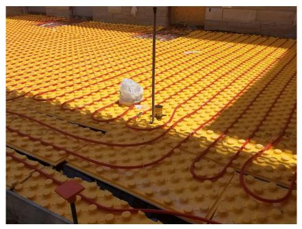
placed 5-6 in (13-15 cm) below the concrete sidewalks, and from there the installers simply snapped the piping in place with pre-made building plastic diamonds inside the boards. In addition to ease of installation, the Creatherm boards also minimize heat loss by preventing heat from travelling into the ground below.
