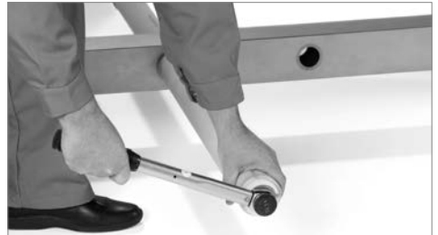
Fig. 4: Installation using torque wrench
