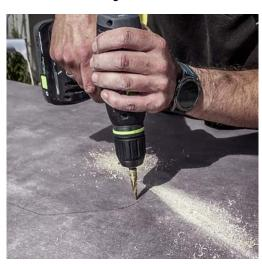
Flexible on-site holes can be drilled easily. REHAU recommends using the following procedure for drilling:
