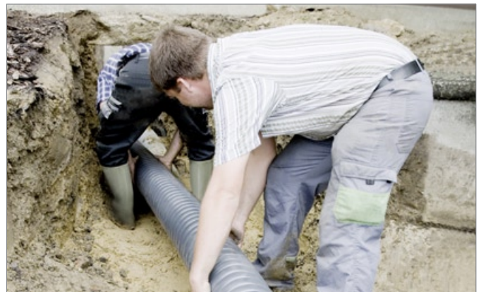
The high degree of flexibility provided by the corrugated casing makes the task of threading the pipe into house connections a lot easier.
