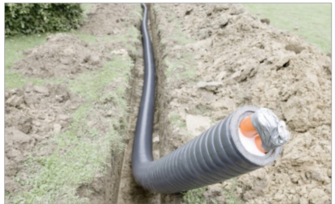
The soft insulation means that the pipe can be laid easily and quickly, with low associated personnel costs.
