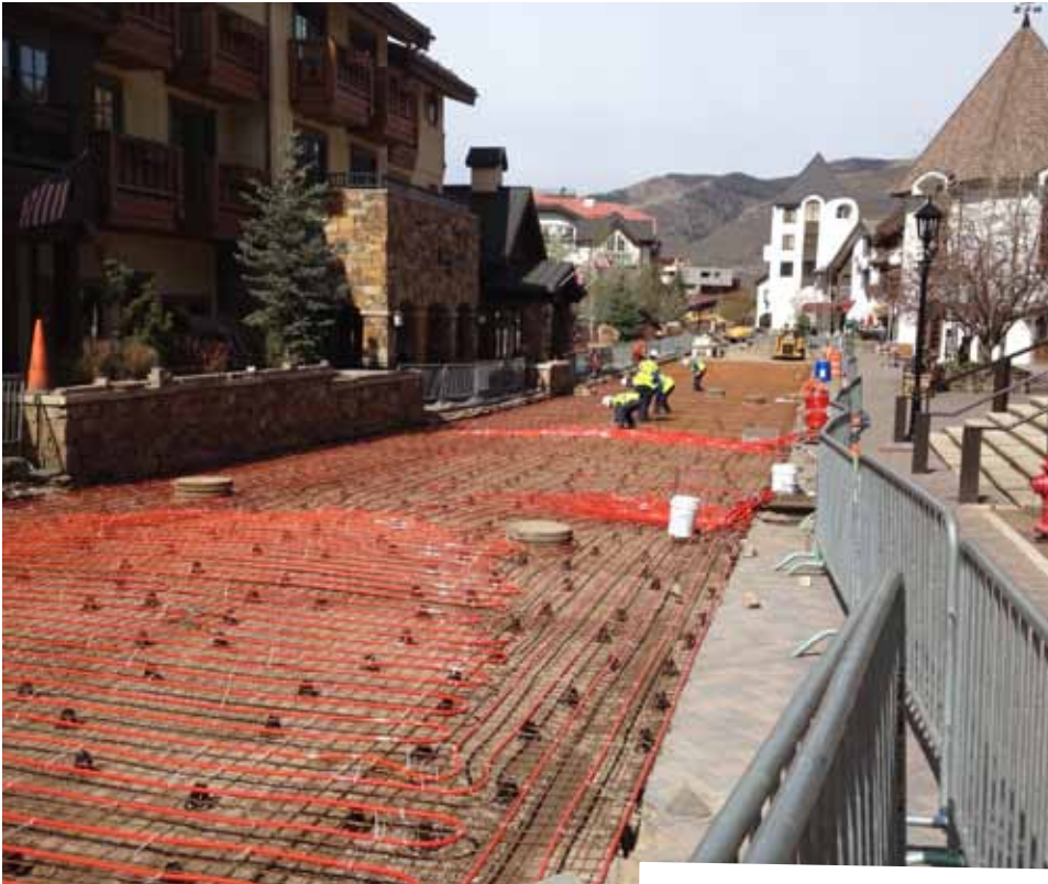
Above: Workers install REHAU plastic pipe for the snow-melt system at the Solaris Residences in Vail, Colo. Inset: The snow-melt application at Solaris won REHAU a Plastic Pipe Institute Building and Construction Division 2011 "Project of the Year" award.
