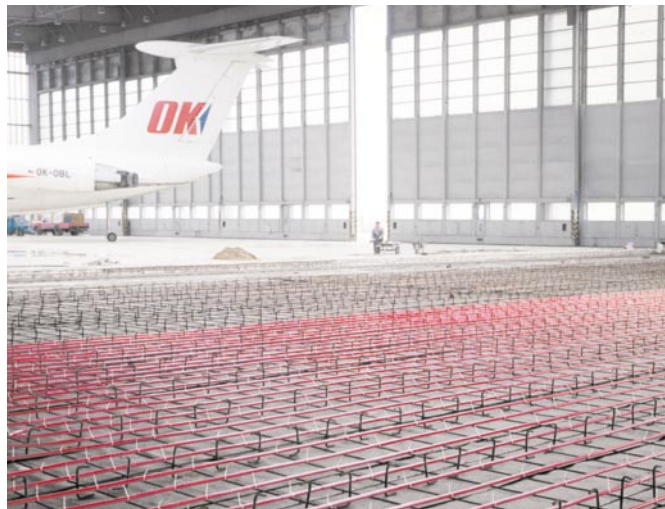
Industrial underfloor heating - a modern heating concept for buildings employed for industrial purposes
