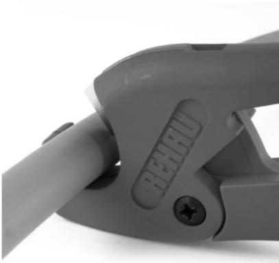
1. Use an approved plastic pipe cutter to cut the pipe to the desired length.
