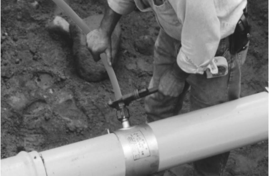
*Fig. 10: Angle MUNICIPEX reclaim pipe 10 to 20° above horizontal at connection to main*
