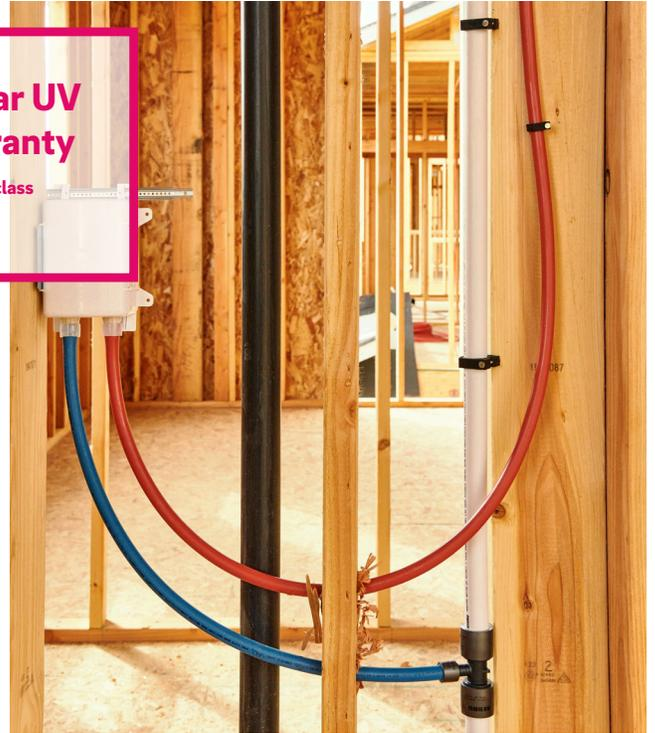
Easily bend RAUPEX instead of using elbows to make directional changes or navigate crowded mechanical chases, saving time on labor and money on fittings.
