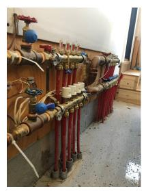
The circuits were connected to 1 in. REHAU PRO-BALANCE manifolds via 1 in. RAUPEX O2 barrier supply and return piping. To accommodate the multiple zones throughout the home, the main level, second level and basement each have two manifolds and the garage has one. "I like how the PRO-BALANCE manifolds go together," Kardumovic said. "Compared to other manifolds I've used, REHAU's manifolds are easier to connect to the pipes and they look very neat."
