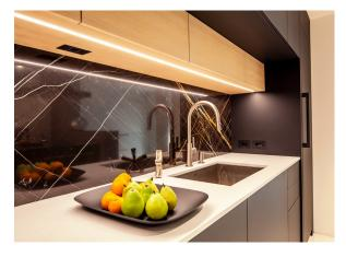
during the permit process. We used LVL engineered lumber to make the wall structurally flat, added generous blocking, insulation and sound proofing, then pre-installed a monolithic backsplash fabricated from a single slab of Sahara Noir marble with no penetrations. We absolutely needed to give Strong Cabinetry a flat substrate to work from."
