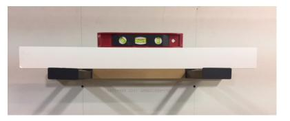
11. Install the foam blocks on each end bracket with the foam surface facing down and the cardboard surface facing up. Place foam blocks only on the two brackets closest to the floating shelf ends.
