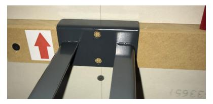
7. With the bracket removed, drill holes in the center of the hole locations. Use a 5/32" or smaller drill bit and drill through the MDF into the wall stud.
