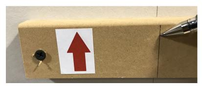
6. Position the floating shelf bracket on the MDF strip so that the bracket holes are centered on the wall stud. Mark hole locations with a pencil or marker.
