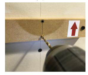
9. Repeat the above step for each floating shelf bracket. You must use the number of brackets specified below, which is based on the length of your shelf. In some cases, this means you may not be required to use all brackets supplied.
