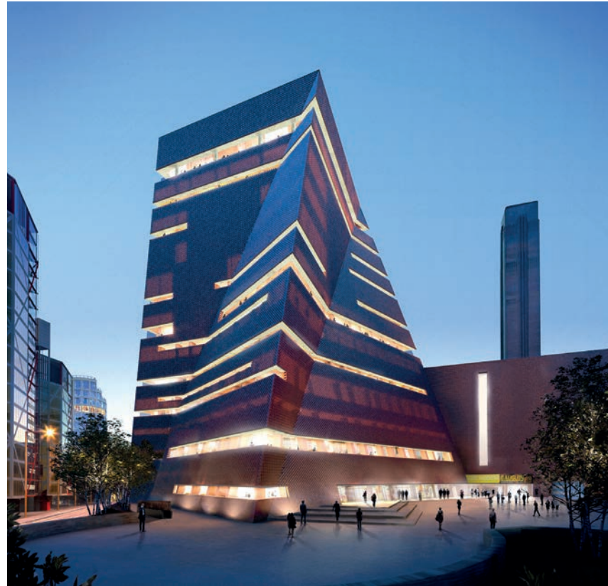
Tate Modern, London Size: 24,000m of pipework in new building extensions Product: TABS
