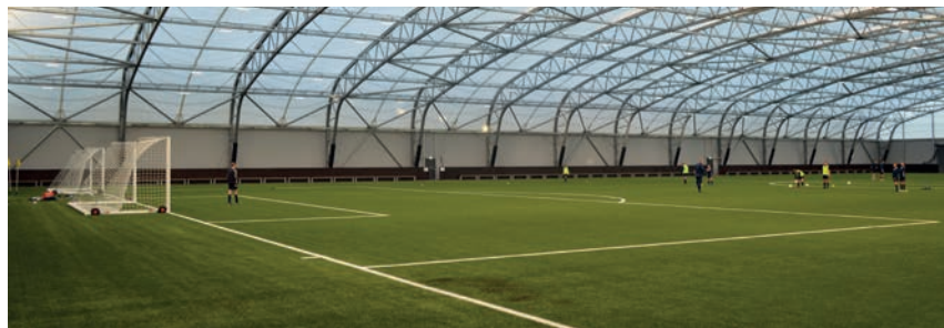
Regional Performance Centre, Dundee Size: Pipe installed between the energy centre and rest of the development Product: RAUTHERMEX pre-insulated pipe
