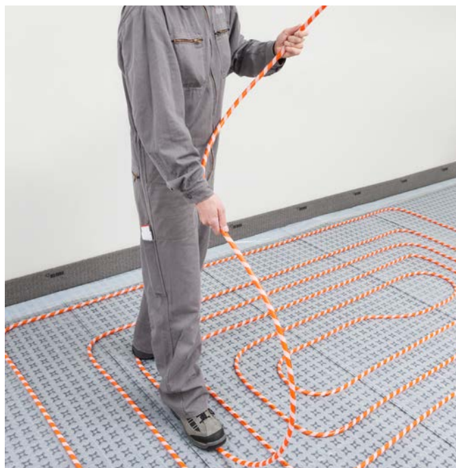
RAUTHERM SPEED plus buisinstallatie
