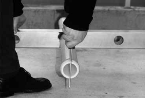
Figure 3: Align with screwdriver 图 3: 用螺丝刀固定住曝气管
