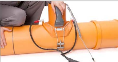
Connect the welding cable to the electrofusion saddle in a load relieved way, enter the welding data, e.g. using a barcode reader, check the display on the welding machine and carry out the welding process.
