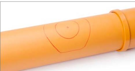
5. Immediately prior to welding, remove the oxide layer completely from the pipe surface in the welding area with a scraper. The marking lines (hatching) must be removed completely after scraping. Swarfs are to be removed. Clean the processed pipe surface and the interior surface of the electrofusion saddle with a special cleaning agent (see stipulations of DVS 2207-11) and unused, absorbent, non-fibrous and non-coloured paper and allow to dry.
