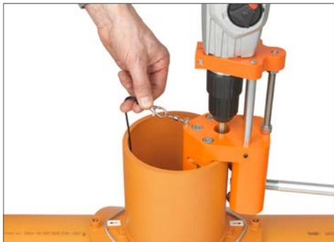
16. Mill out the opening in the main pipe by turning the milling fixture clockwise. If necessary, pass over the starting point with several left/right turns in order to obtain a clean cut. Remove the swarfs in the milling area.
