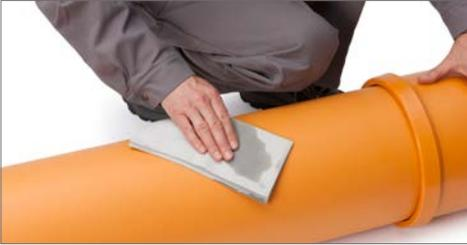
3. Mark the welding area using hatching.
