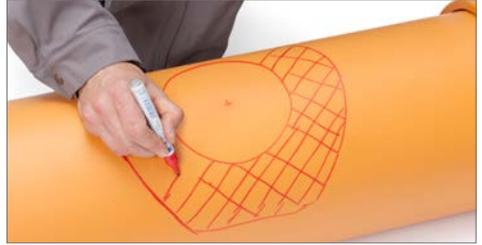
2. Place the electrofusion saddle in the designated position on the pipe, trace the exterior and interior contour of the saddle and mark the centre of the saddle outlet.
