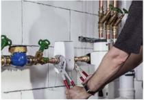
Have the RE.GUARD water control device installed by an expert, ensuring it is positioned after the water meter and before the house filter. Done!
