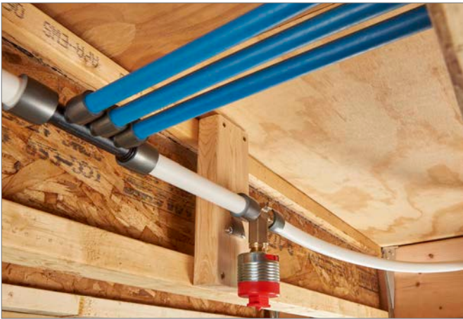
Fig. 6.2: Domestic cold water plumbing connection
