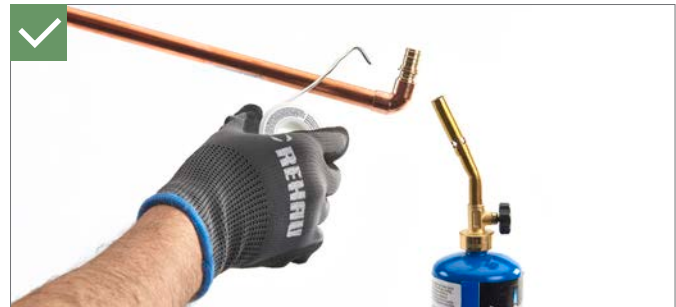
Fig. 7.22: Solder prior to making EVERLOC+ connection
