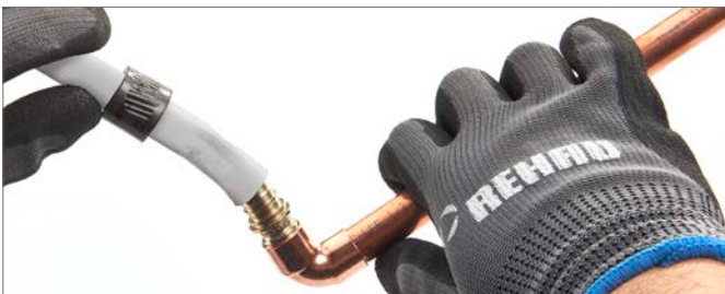
Fig. 5.10: Removing pipe from LF brass fitting
