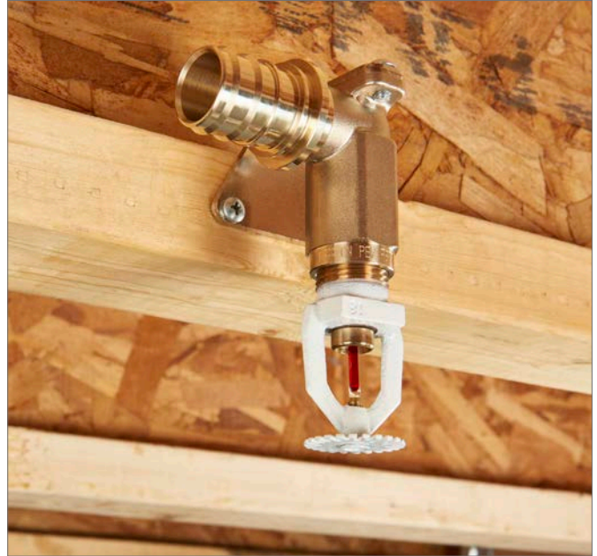
Fig. 7.7: Recessed pendant sprinkler mounting example
