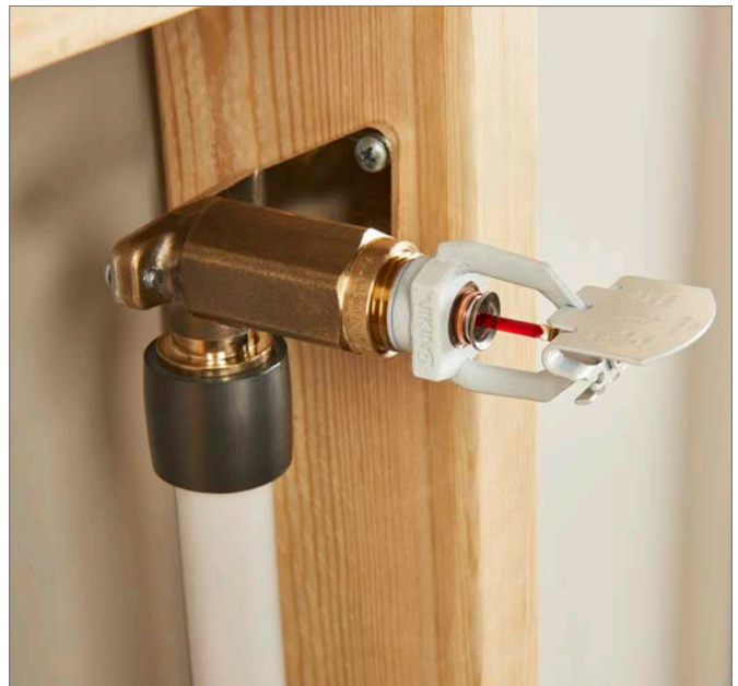
Fig. 7.9: Horizontal sidewall sprinkler mounting example
