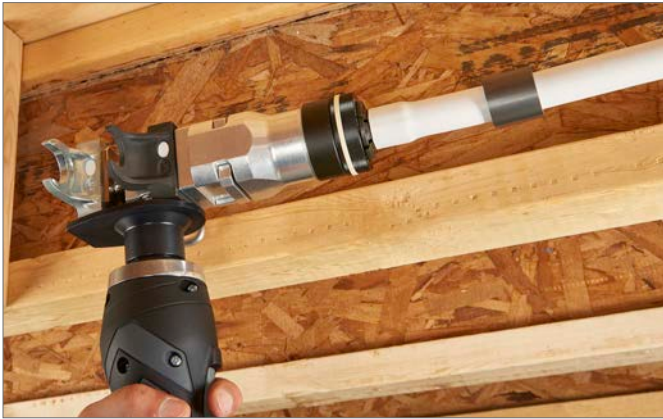
Fig. 7.10: Expanding RAUPEX white UV shield pipe
