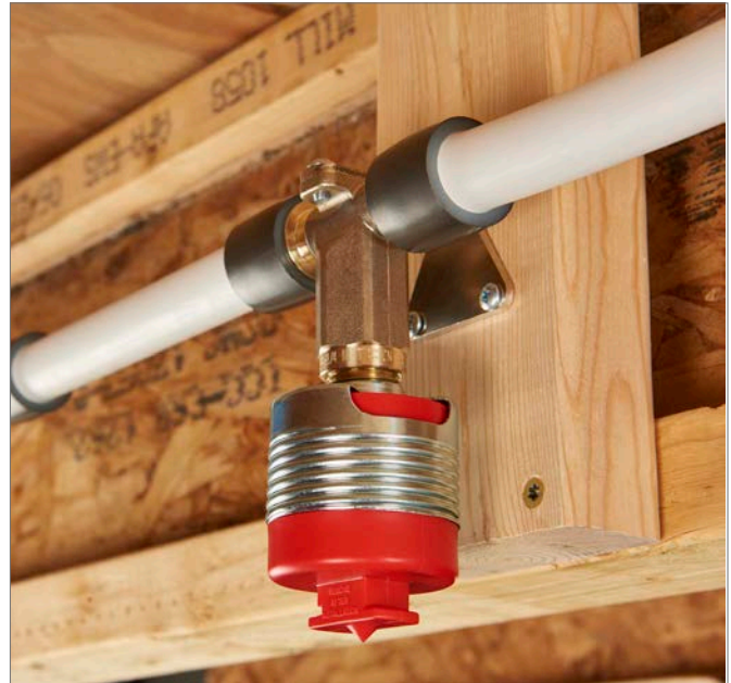
Fig. 7.3: Flat plate pendent concealed sprinkler mounting example
