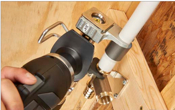
Fig. 7.11: Compressing EVERLOC+ sleeve
