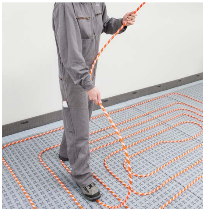
Installation du tuyau RAUTHERM SPEED plus
