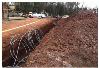
Just now coming into its own in geothermal applications, PEX has been used as geothermal ground loop piping in Europe for more than a decade.
