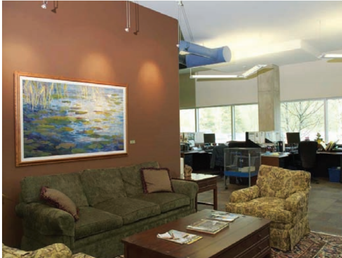
Specifiers integrated the engineering functionality of an exposed concrete radiant-cooled ceiling with the architectural vision of exposed ductwork and drop lighting to provide a collaborative feel within the interior space at Earth Rangers Centre (ERC) in Woodbridge, Ontario.
