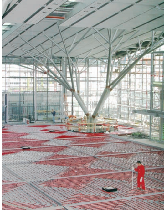
These images show the radiant pipe layout at the Stuttgart Airport
