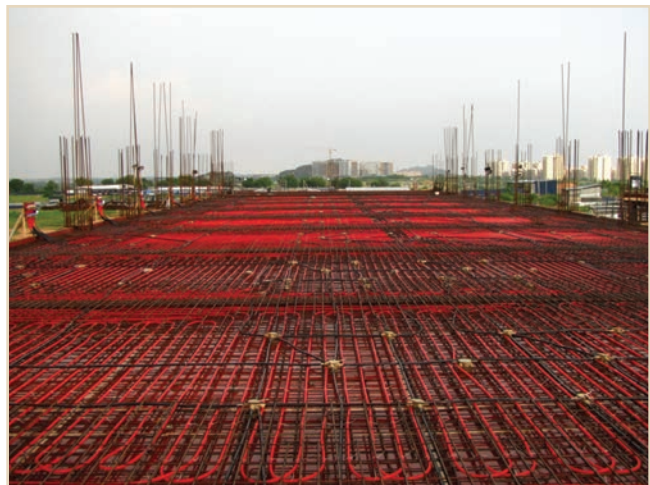
FIGURE 6: Radiant slab system before concrete pour.
