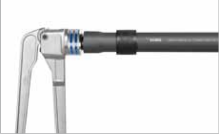
1. Expand the pipe
