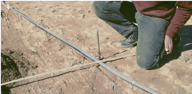
Fig. 19: Stake pipe in place
