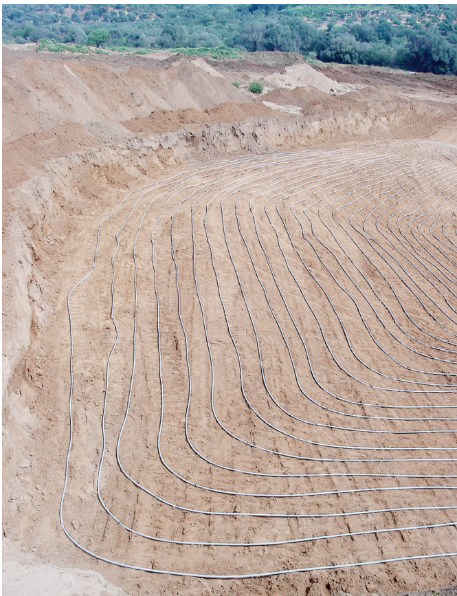
Fig. 20: Pressure test system before burial
