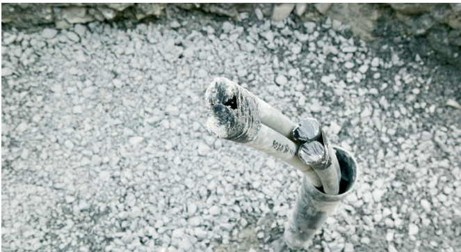
Fig. 23: Compacting the annular gap with grout
