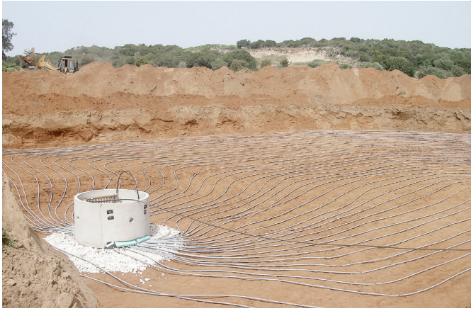
Fig. 18: Uncoil pipe
