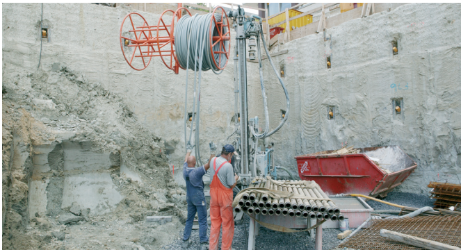
Fig. 22: Fastening the U-bend weight
