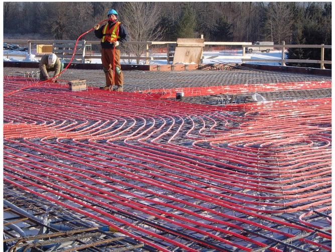
The system's cooling function employs concrete slabs that are actively cooled to approximately 64° F (18° C) overnight using circulating water from a cooling tower or geothermal wells. The slabs warm up slightly during the day as they absorb heat from the space. This technique provides much of the building's cooling energy on an average day and significantly cuts electricity use.
