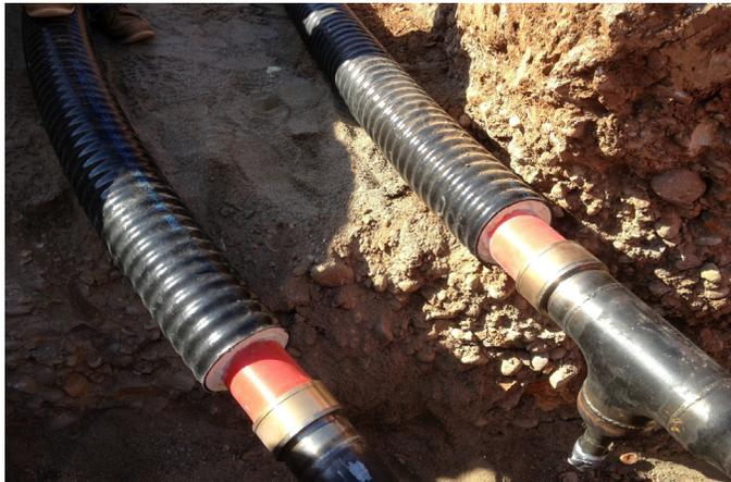
The new administration building at Miramar College comprises 17,000 ft<sup>2</sup> (1,579 m<sup>2</sup>) of new construction at the north end of campus. Plans originally called for installing a heating and cooling system similar to the campus's existing system, which distributed hot and cold water through steel pipe. After consulting with REHAU representatives, however, Southland Industries, the project engineer, decided to use REHAU INSULPEX pre-insulated PEXa pipe.
