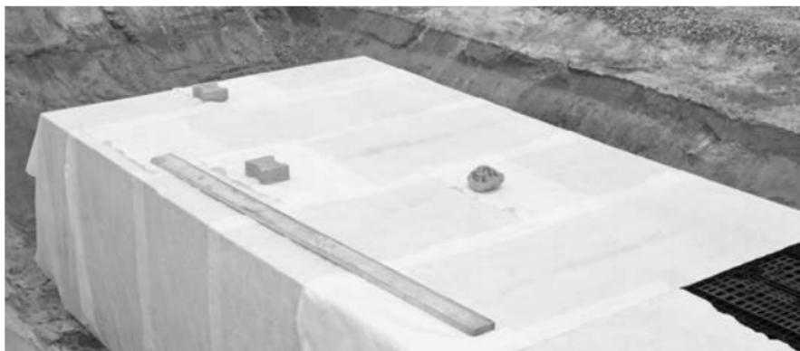
*RAUSIKKO Box with geotextile filter*
