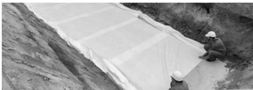
*Prepared trench with RAUMAT geotextile filter*
