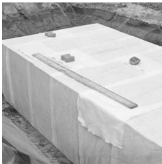
RAUSIKKO Box tank with RAUMAT geotextile filter
