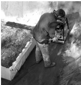
Compacting the work area
