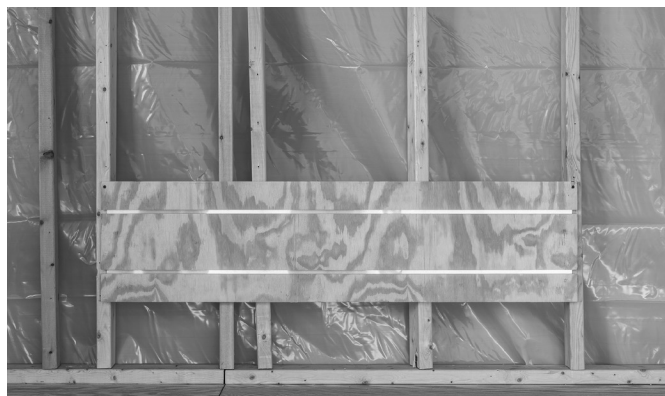
Fig. 12: Install header row for wall installation
