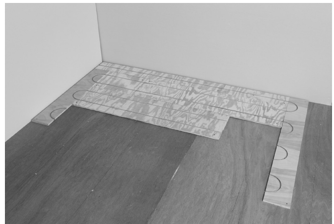
Fig. 7: Fill-in with double groove panels, staggering joints
