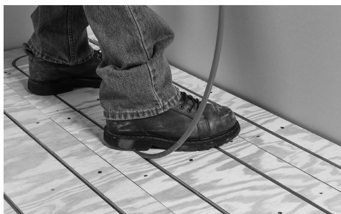
Fig. 16: Snap pipe into groove with silicon
