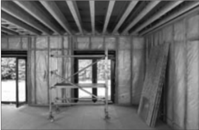
Fig. 2: Underside of joist space construction
