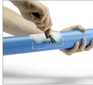
Fig. 54 2. Using the manual scraper, remove the sheathing from half the diameter of the basic pipe between the markings. The chip thickness should be approx. 0.2 mm.
