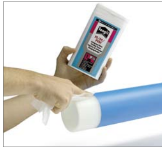
Fig. 43 5. The scraping area must be free of dirt and oil. Clean the area with an adequate amount of Tangit cleaner, and subsequently allow the cleaning agent to completely evaporate.
