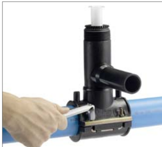
Fig. 56 4. Attach the tapping clamp
