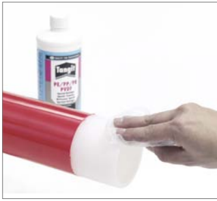
Fig. 95 The scraping area must be free of dirt and oil. Clean the area with an adequate amount of Tangit cleaner, and subsequently allow the cleaning agent to completely evaporate.
