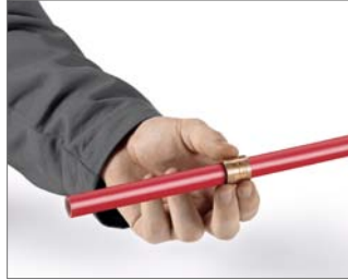
Fig. 12 2. Push the compression sleeve over the pipe end. The internal chamfer must face the pipe end.
