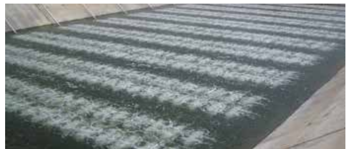
EJIP WWTP (Indonesia)
