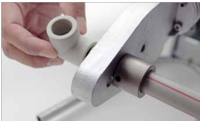
Fig. 8-6 Heat the pipe and fittings
