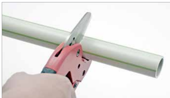
Fig. 8-4 Cut the pipes
