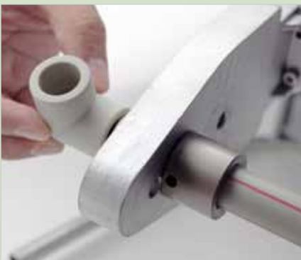
1 Heat the pipe and fitting
