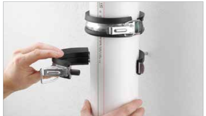
Fig. 7-16 Closing supporting bracket.
