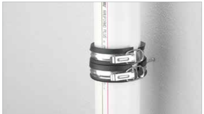
Fig. 7-17 Fully installed sound-dampening bracket.
