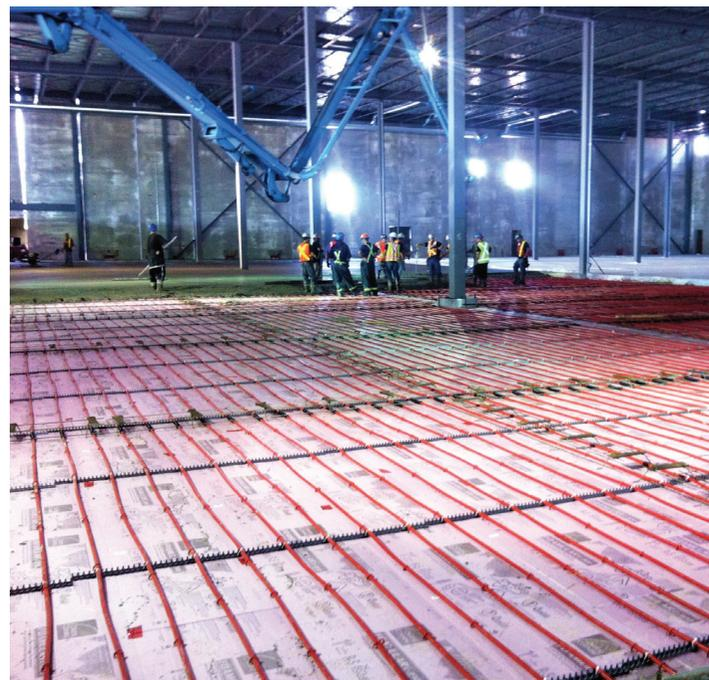
**ABOVE:** At Ontario-based Belmont Farm Supply, a REHAU radiant heating system keeps floor temperature between 57° F to 60° F to protect fertilizer and other products being stored.
