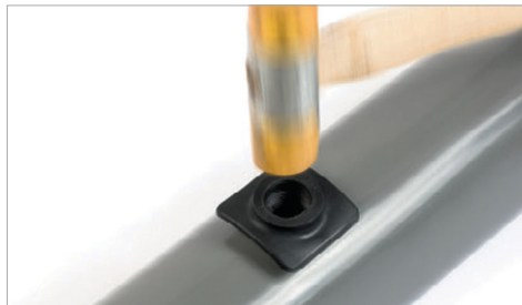
Figure 28: Grommet installation into a 32 mm hole using a rubber mallet 图 28: 把双承接头安装在一个直径为32mm的孔上
