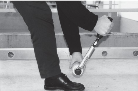
Figure 4: Check maximum torque with torque wrench 图 4: 用扭力扳手上紧
