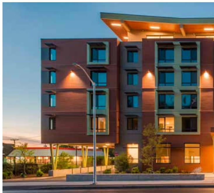
multiple chambers, engineered compression-seal technology and high-quality uPVC formulation, allowing these tilt-turn windows to be up to 45 percent better than thermally broken aluminum.
