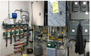
From the boiler room, all manifolds were supplied with 11/2-in. RAUPEX O<sub>2</sub> barrier supply lines, he adds. The longest supply lines were nearly 300 ft (91 m) from the heat source.
