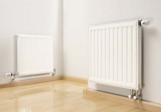
Fig. 25-1 Radiator connection from skirting
