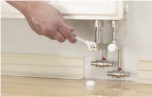
Fig. 25-12 Tighten the manifold union firmly
