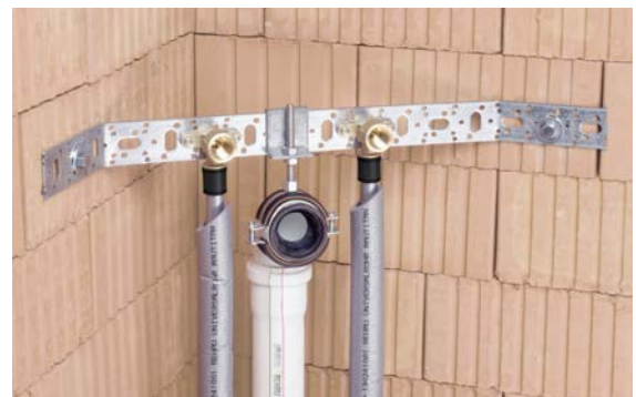
Fig. 10-3 Installation example: Installation rail
