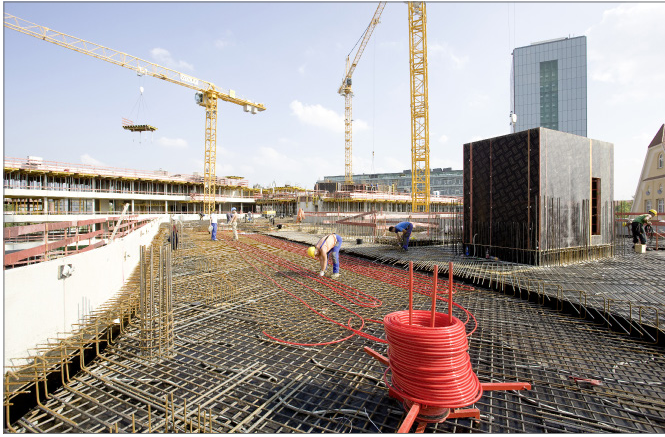
Fig. 2-3 REHAU CCT installed on site
