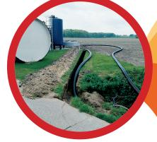
Open trench – this is the most common technique. Narrow trenching can be used if the installer can work safely to make any joints. Damage to the jacket pipe from poor handling can be repaired using a suitable repair set available from the manufacturer.
