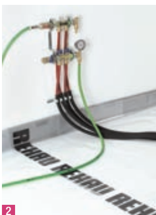
2 Flushing the circuit
