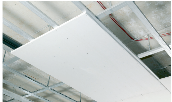
Fig. 2-5 Installed ceiling element
