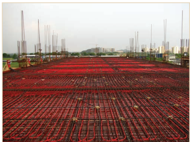
FIGURE 6: Radiant slab system before concrete pour.
