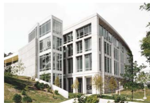
Headquarters in Leesburg The administrative center in Leesburg, Virginia, is located near Washington D.C. This headquarters serves United States, Canada and Central America.
