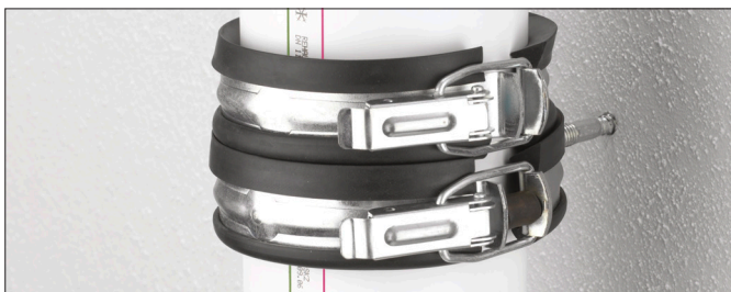
Fig. 3-6 Fully installed acoustic bracket
